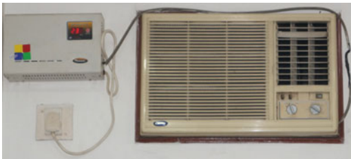
Window air conditioner
